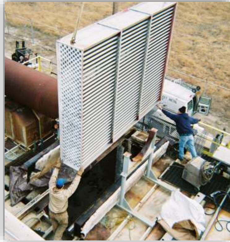
Catalytic & Recuperative: Metal Heat Exchangers 60-80% Efficient
