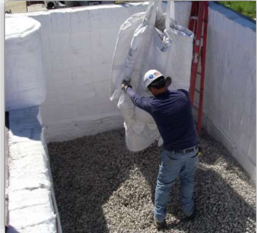
Regenerative Thermal: Ceramic Heat Recovery Media 95-97% Efficient
