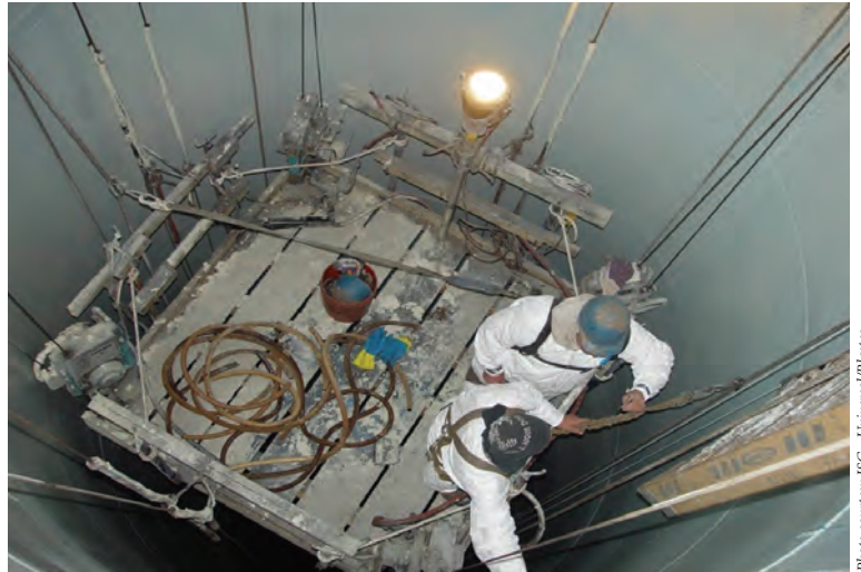
A vinyl ester resin lining is applied in a smoke stack.
